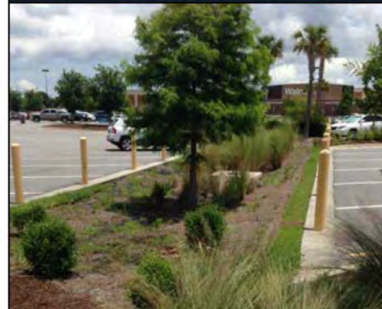
Parking Lot Drainage Swale
