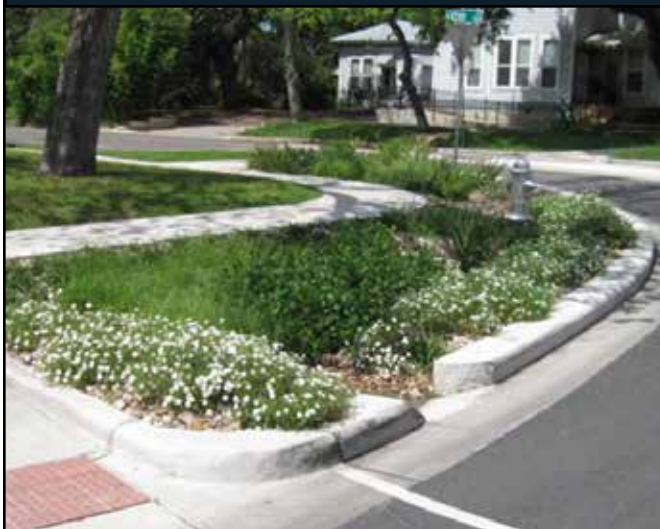
Parking Lot Drainage Swale
