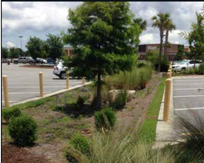
Parking Lot Drainage Swale
