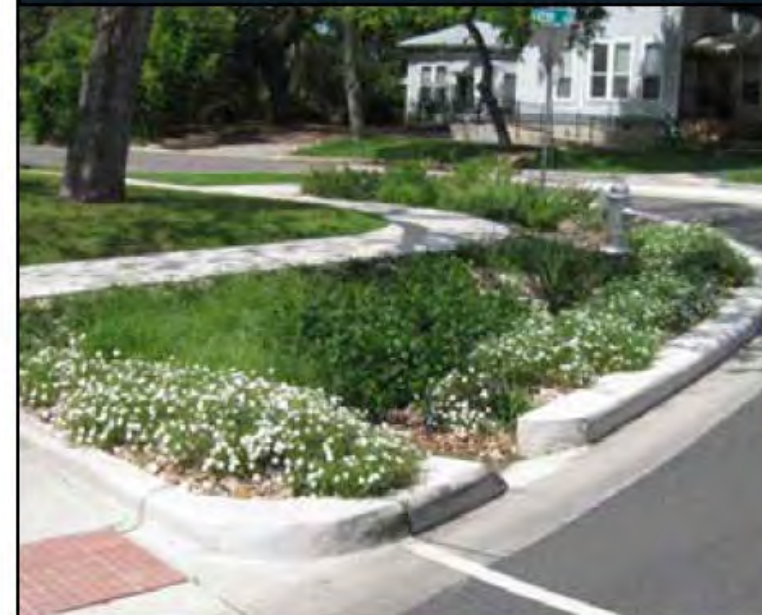
Parking Lot Drainage Swale
