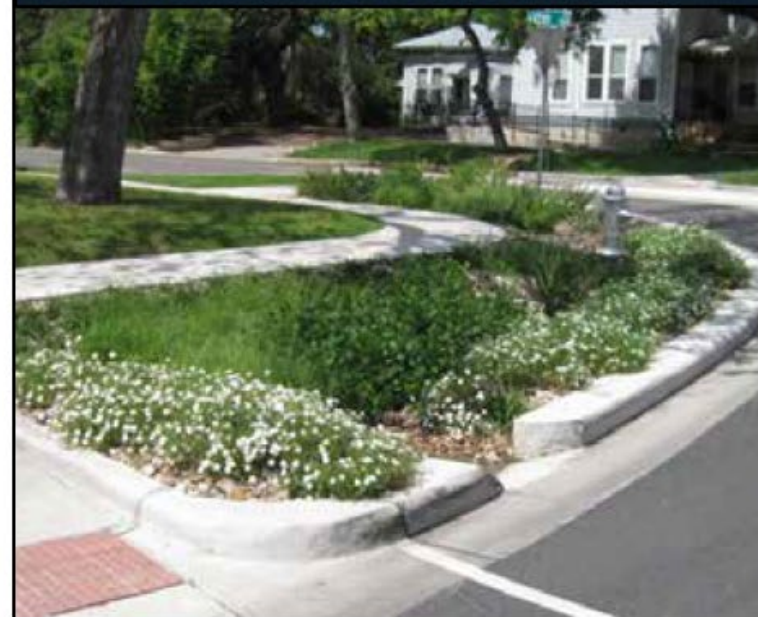
Parking Lot Drainage Swale
