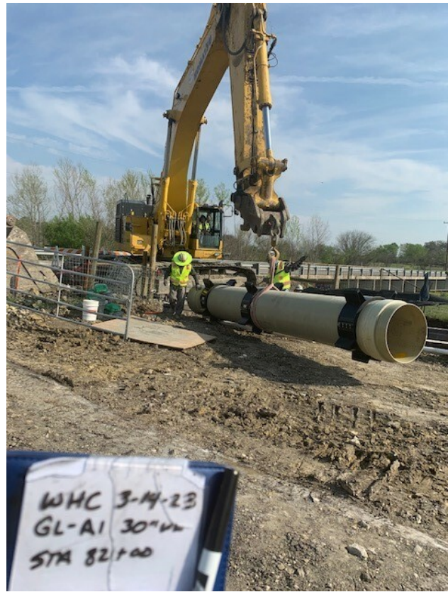
30" pipe with spacers to be inserted in casing below Trainer Hale Road
