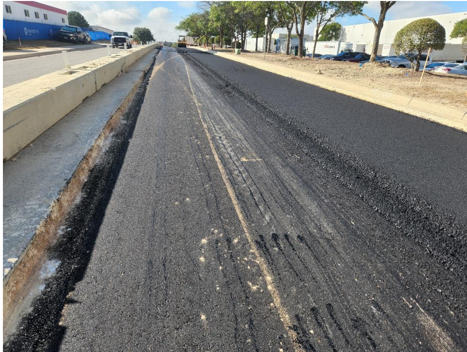
Second Layer of Pavement
