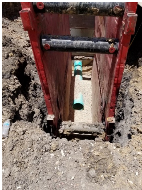
Starting Pipe Installation
